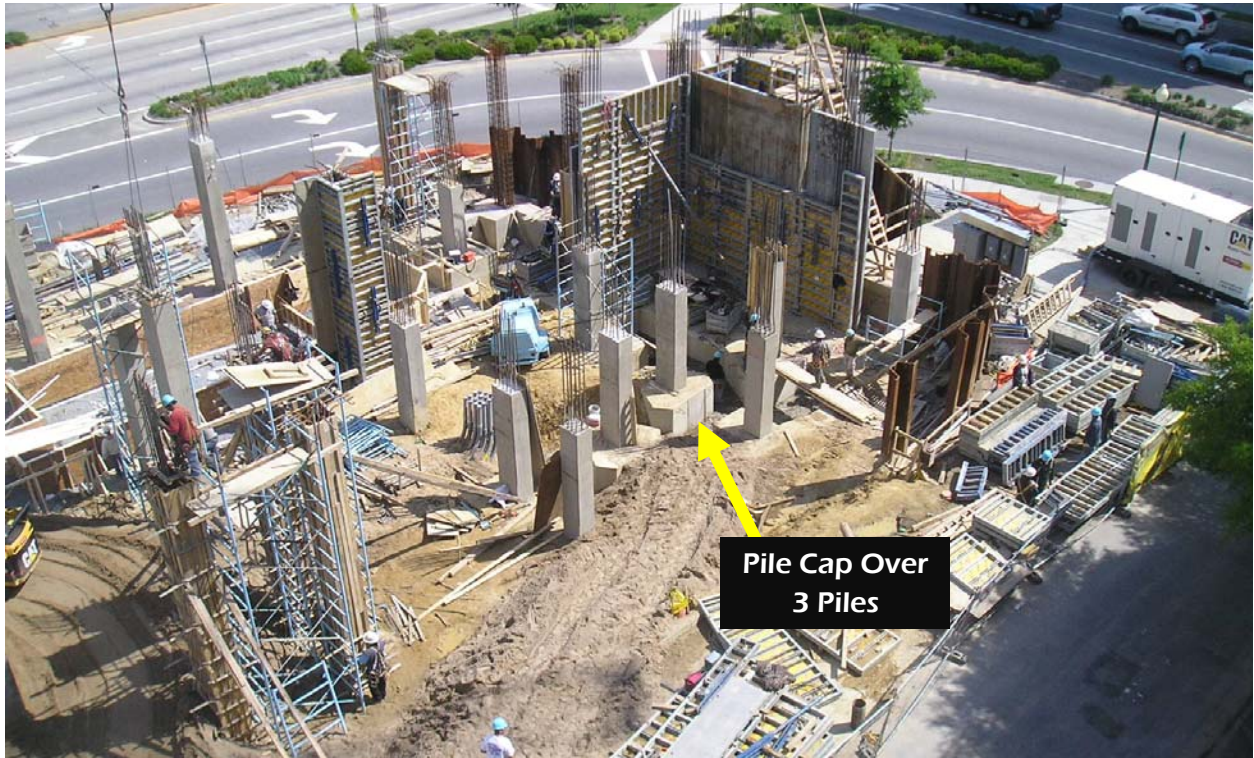
(FIGURE 16) Foundations & 1 st Floor Columns under Construction
