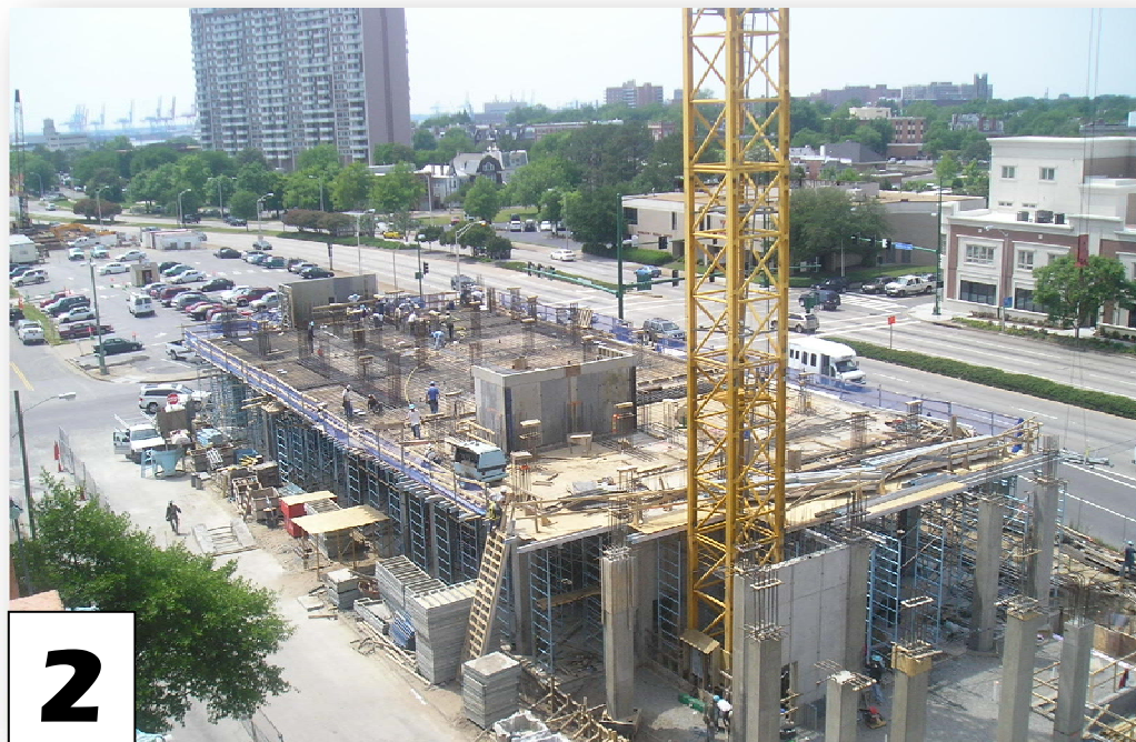
(FIGURE 4) Aerial View from NW Looking SE
